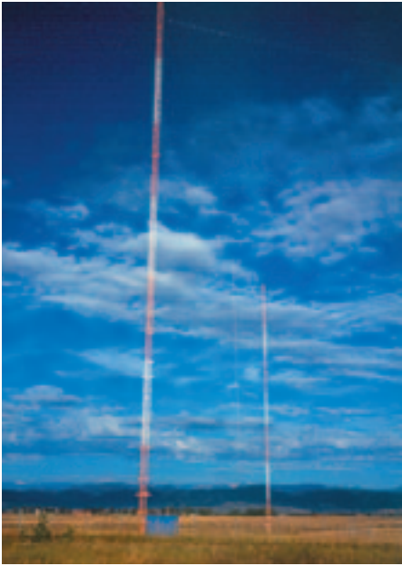
Figure 2.2. WWVB Antenna Towers
